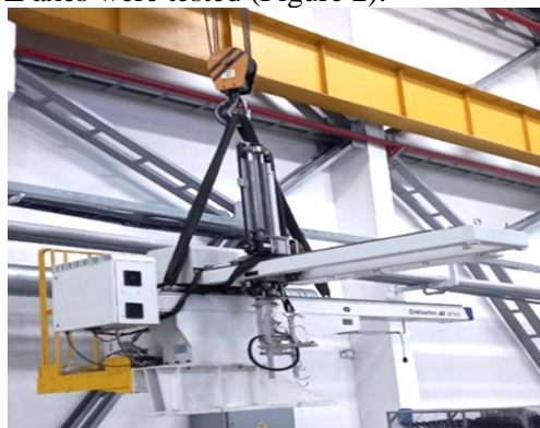
Figure 2. Process of installing the robot onto the machine using the prepared fixture
